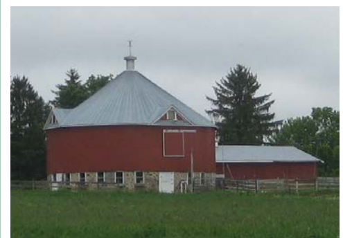
Another classic round dairy barn. It is along STH 54 in Waupaca County and is easily visible from the highway. Imagine if this gem disappears from the landscape? We need to do more to help farmers and other property owners preserve and protect these wonderful icons of Wisconsin!
