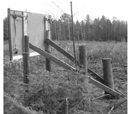
Left - Structural repairs using treated lumber to a non-conforming billboard.
